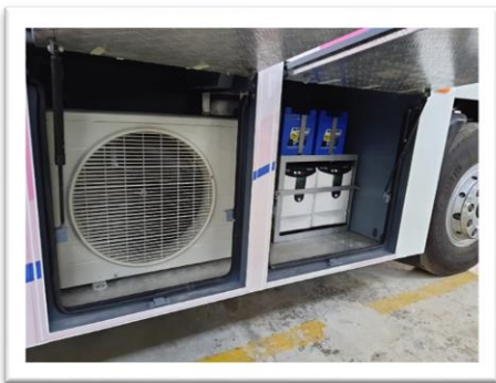
Power inverters and AC Unit
