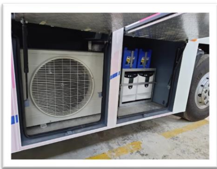
Power inverters and AC Unit
