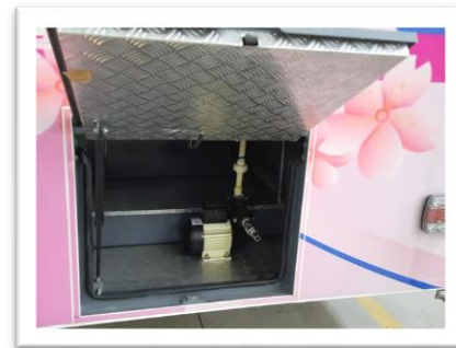
Water pump for the overhead water tank
